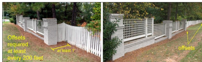
Figure 5.5.G: Fence and Wall Offsets
